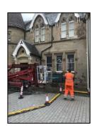
The Mining Art Gallery in Bishop Auckland required targeted paint removal to the ground floor and first floor of the building. Our access lift enabled us to reach the specific areas without requiring scaffolding and allowed us to complete the job in a single day. With the help of paint-rid the DOFF removed the areas of paint quickly and sensitively.
