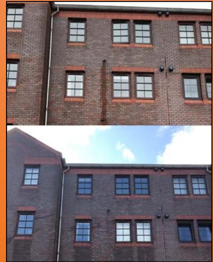
The removal of ferrous staining caused by a leaking downpipe on Orchard Brae
